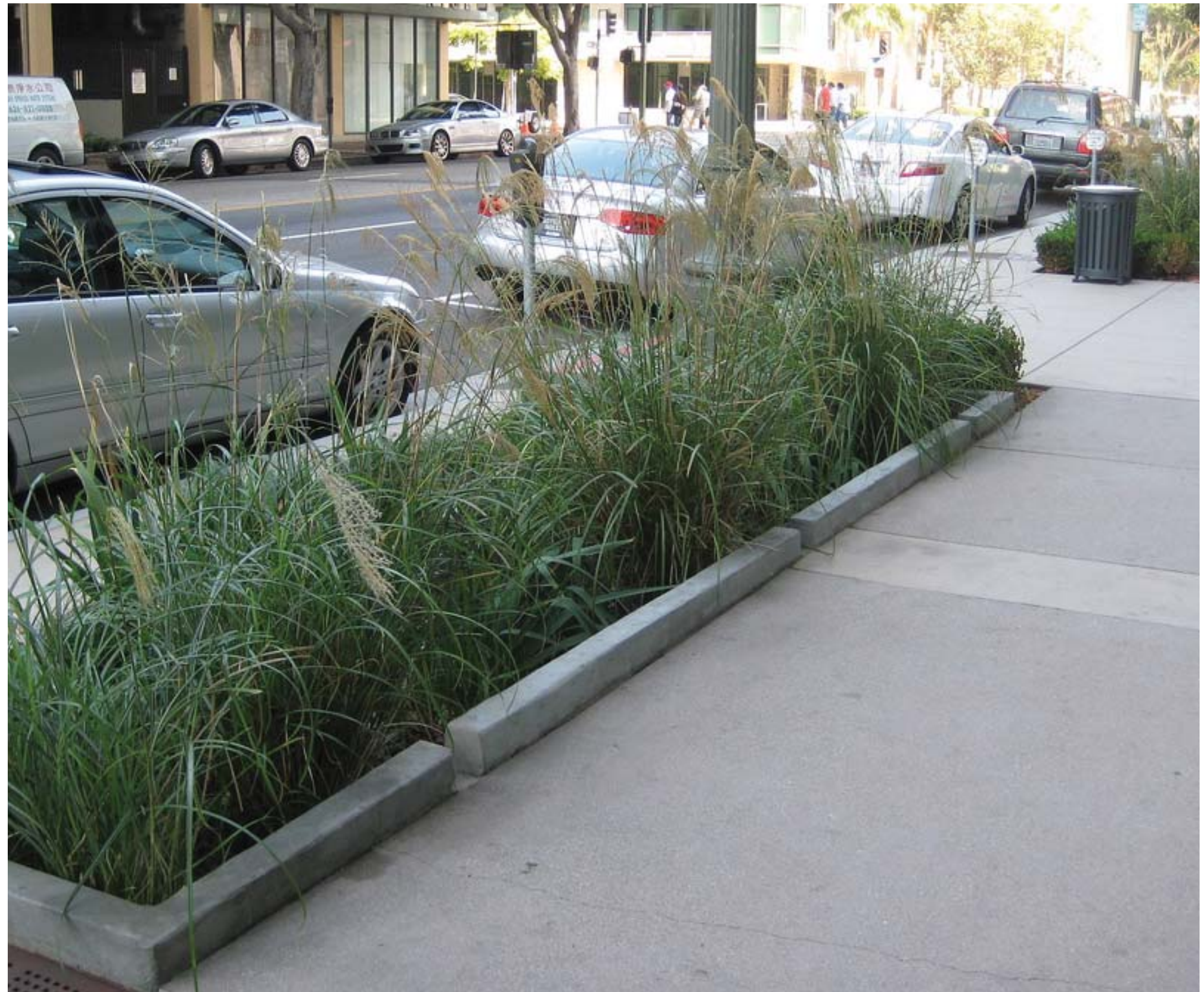
On street storm water planters - Portland, USA
